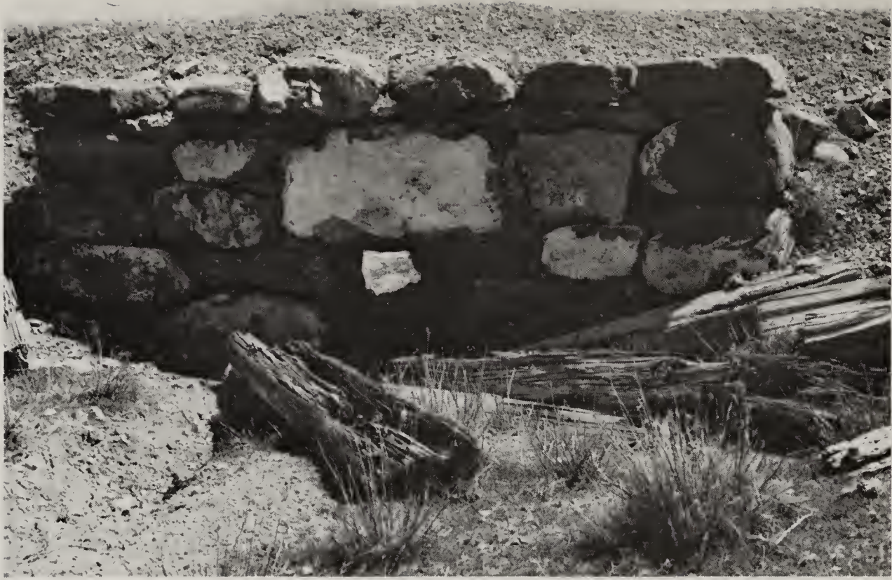
Figure 102: Stone box culvert (BLM photo)
